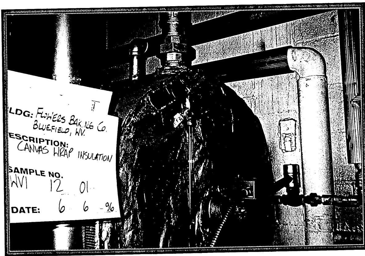
Homogeneous Area Number: 12 Description: canvas wrap insulation on condensate return tank
