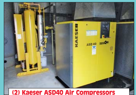
(2) Kaeser ASD40 Air Compressors
