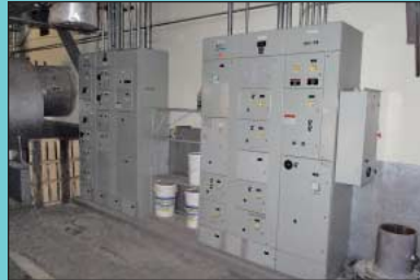
**Air Compressors, Controls and Electrical
