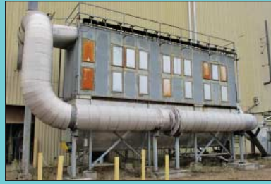
**Dust Collector, 53 Ton Storage Silo, 5.3M BTU/Hr. Air Heater, Blowers
