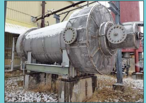
Process Combustion Corp 400MM BTU / Hour Industrial Air Heater
