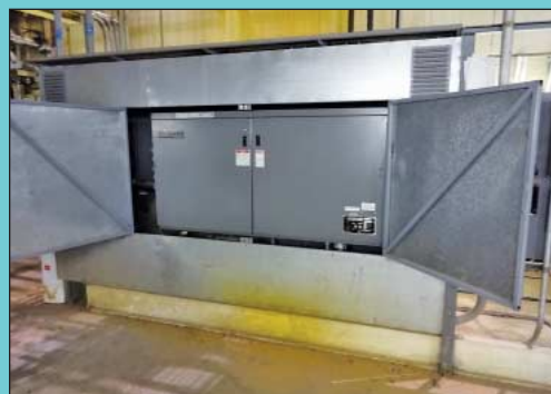
60 Ton (Approx.) Mcquay Model WHR060D Chiller System
