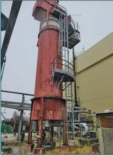
102" Dia. x 30' H (Approx.) American Schack Co. Indirect Fired Metallic Air Heater
