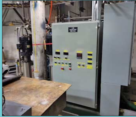
Skid Mount Pump Station with 25 HP Pump and PLC Controls
