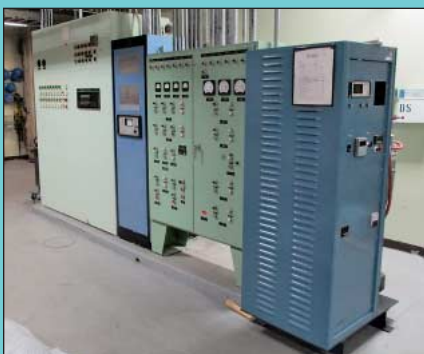
Various Control Panels
