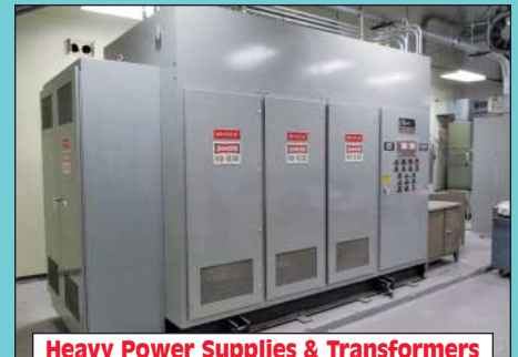
Heavy Power Supplies & Transformers
