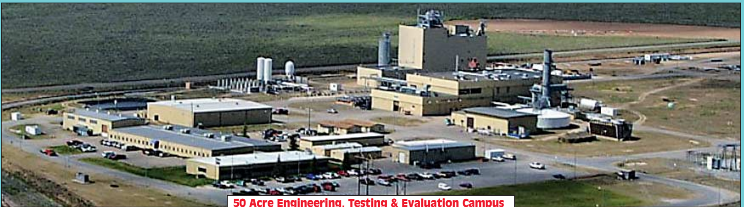
50 Acre Engineering, Testing & Evaluation Campus
