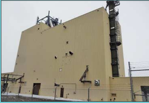
Industrial Minerals Processing Plant
